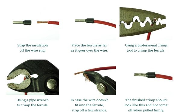
Figure 2 Crimping the wire end ferrules.
