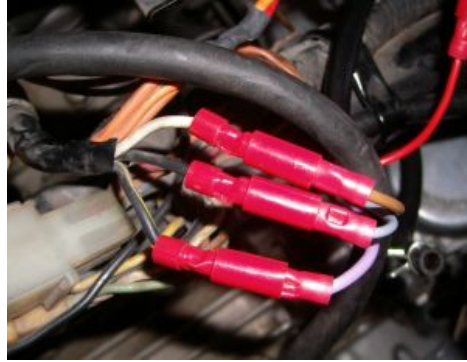
Figure 5 Coil cable connection.
