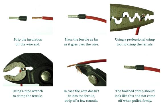
Figure 4 Crimping the wire end ferrules.
