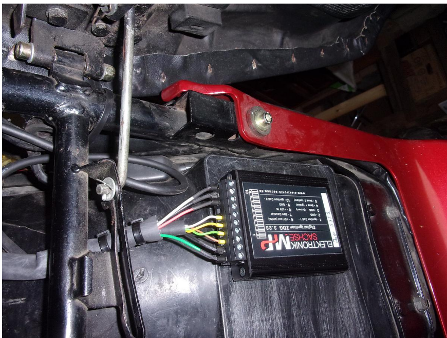
Figure 3 Ignition box mounted under the seat.
