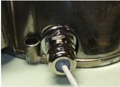
The cable gland with adapter.
