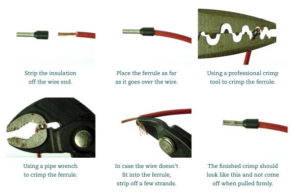
Figure 2 Crimping the wire end ferrules.
