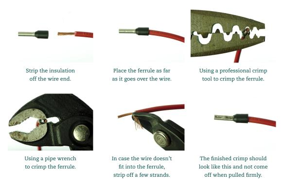
Figure 2 Crimping the wire end ferrules.
